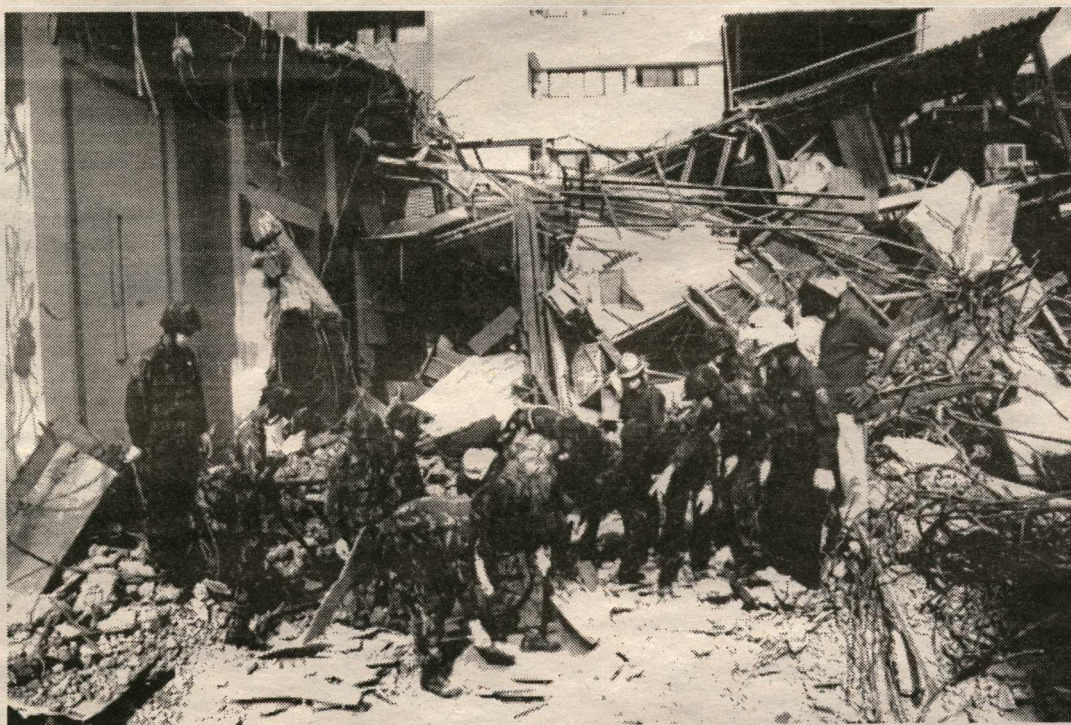
Soldiers and workers rush to help those trapped underneath the rubble of this leveled building. The earthquake measured 7.6 on the Richter Scale and ripped through Taipei.
