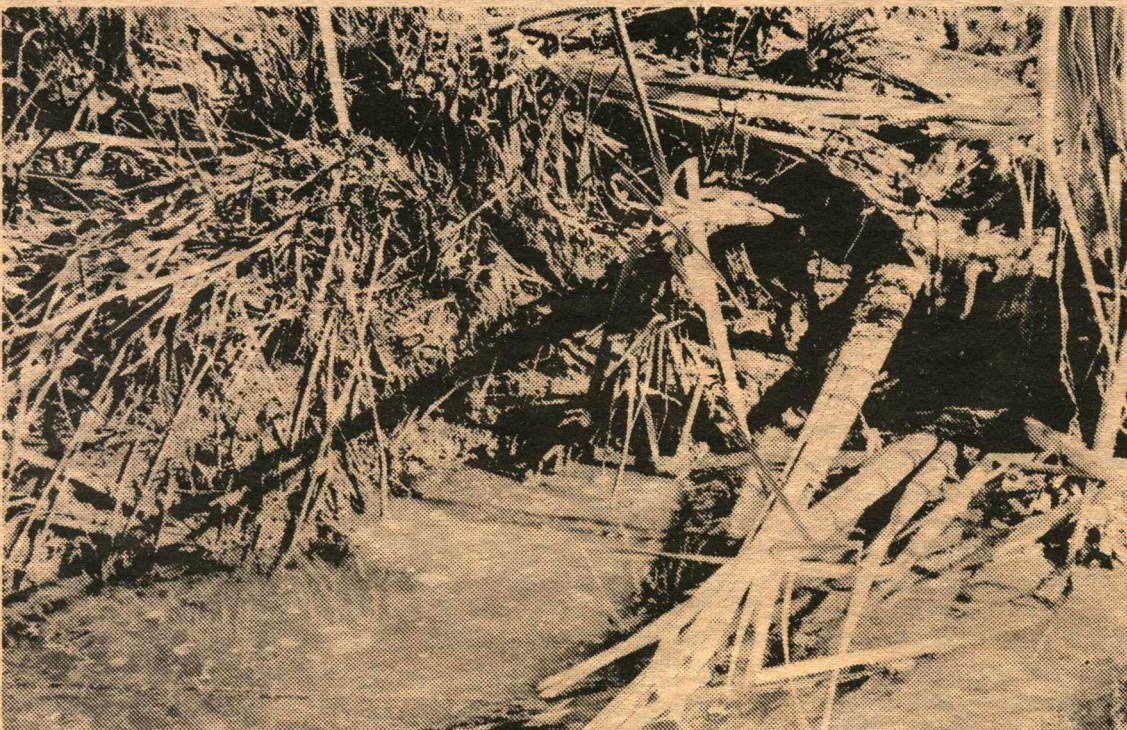
A large amount of sewage, recently discovered to be issuing from Saga's facilities, has been flowing into the Elijah waterway near the Olsen apartments. The problem was eliminated over spring break.
