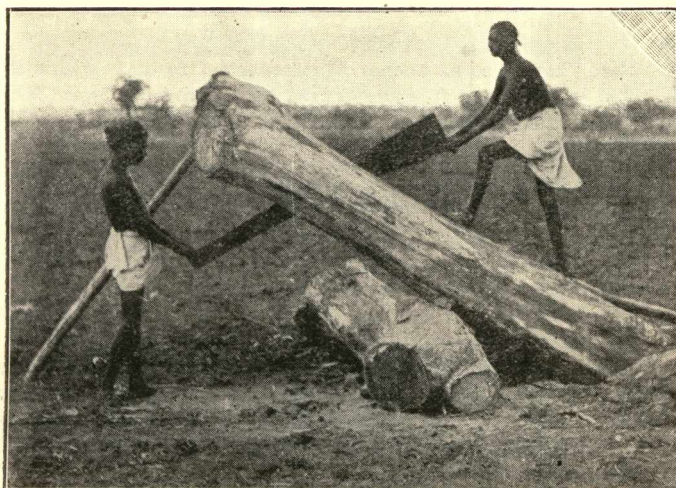
Sawing lumber for construction of a house in Western India.
