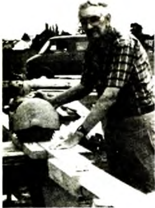
Forrest Buerer, age 66, sawing a length of timber for the Church of the Nazarene Community Hall in Hamilton.
