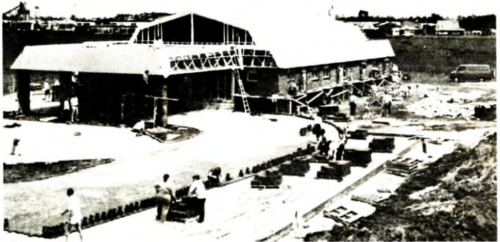
The new Nazarene church hall at Pukete, New Zealand, under construction
