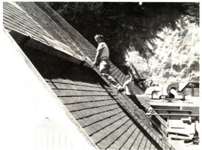
First Church getting new roofing
