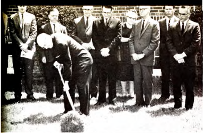
1 Breaking ground for a $48,000 educational building addition to the First Church of the Nazarene of Alexandria, Virginia. District Superintendent V. W. Littrell lifts the first shovel of earth; while looking on, from left to right, are John Danner, E. L. Yingling, and James A. Benton, trustees; Evangelist S. P. Fox; Pastor A. V. Mountford; Mrs. C. A. Goad, charter member; Kemp R. Rush, First Federal Savings and Loan Association of Alexandria; Jess W. Gentry, Sunday school superintendent; and Claude S. Burtnette, Jr., contractor.
